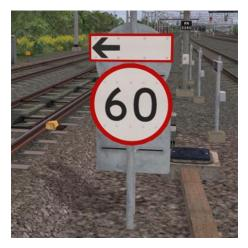
These signs display the permissible speed in miles per hour applicable to the section of line beyond the sign up to the commencement of any subsequent permissible speed section.
