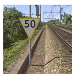
These signs provide advance warning of a reduction in permissible speed ahead. Permanent AWS Ramps (Automatic Warning System) are often installed in conjunction with these signs. In these cases the driver must cancel the AWS warning when triggered on approach to these signs. See safety systems section of this manual.
