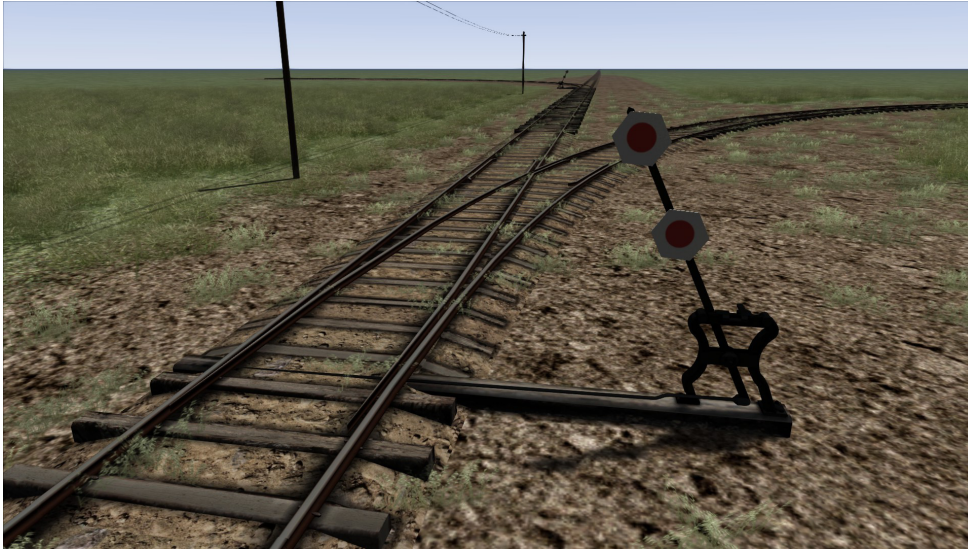
Example 2: Track diverging to the right - thrown switch has the lever pointing left.
