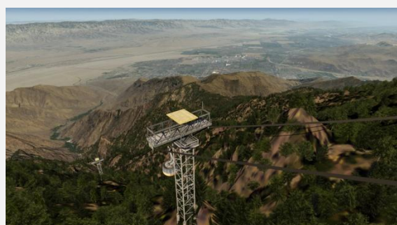
One of the helipads found along the Aerial Tramway
